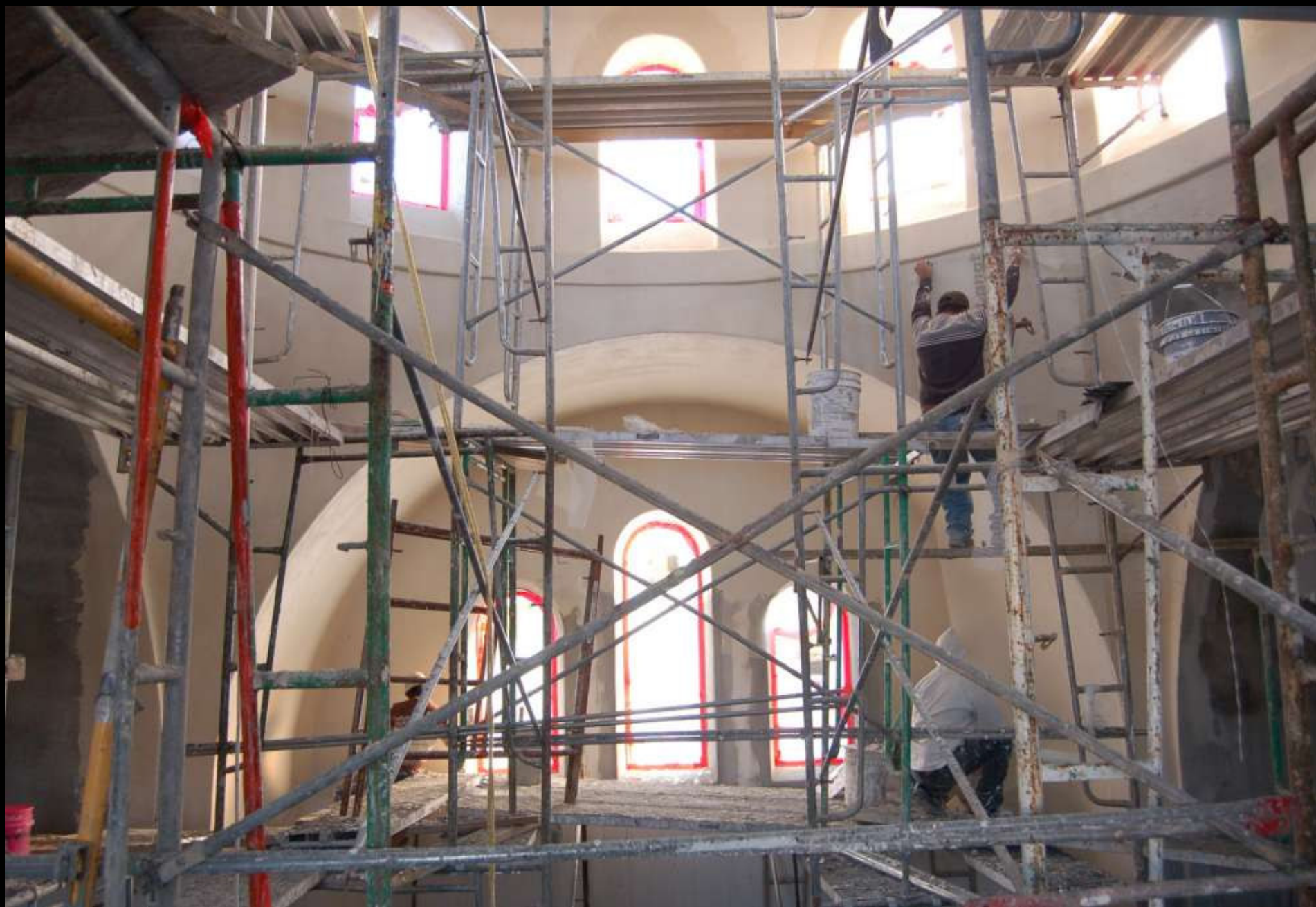
Plastering the interior January, 2008
