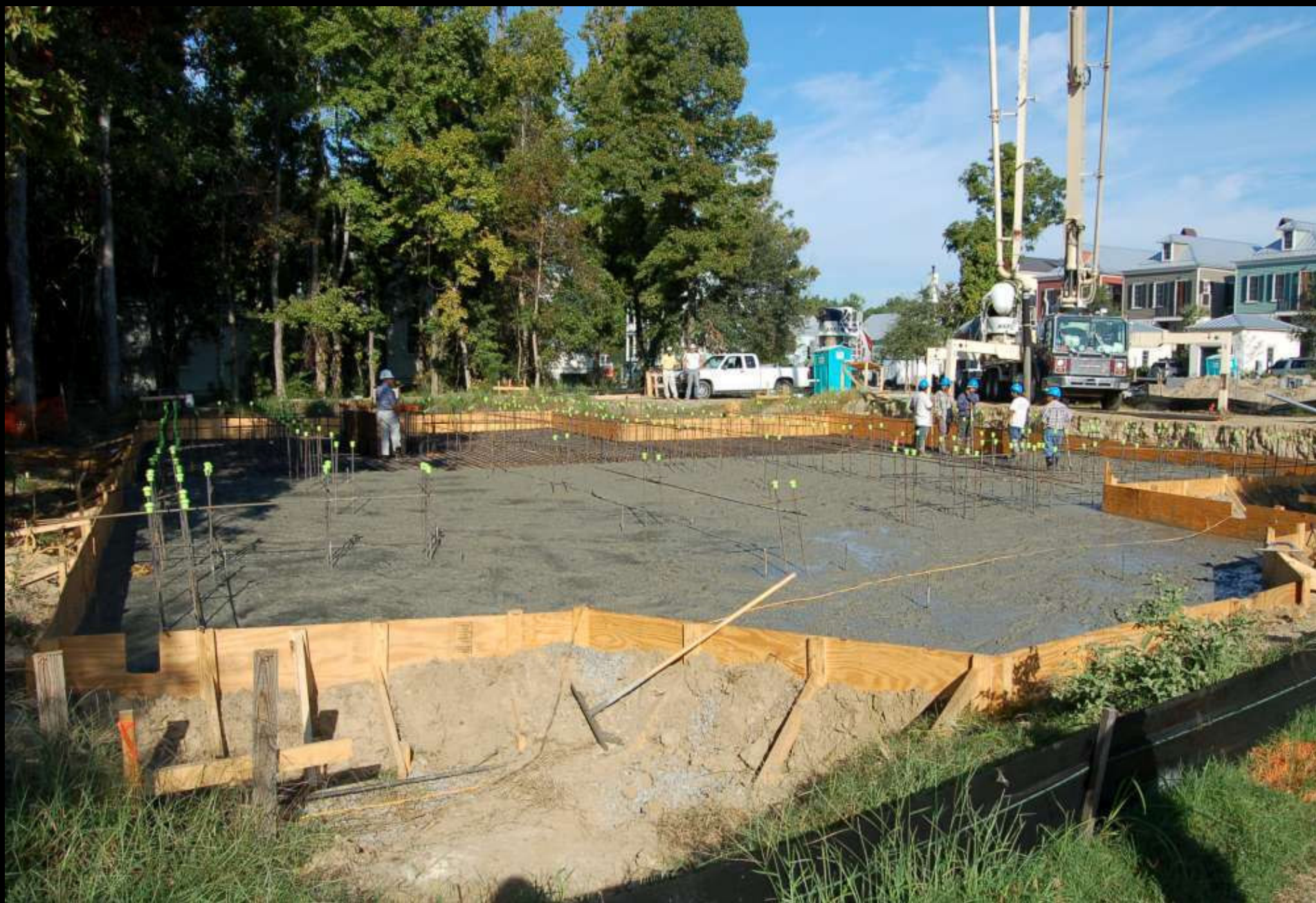
Pouring the foundation slab October, 2006
