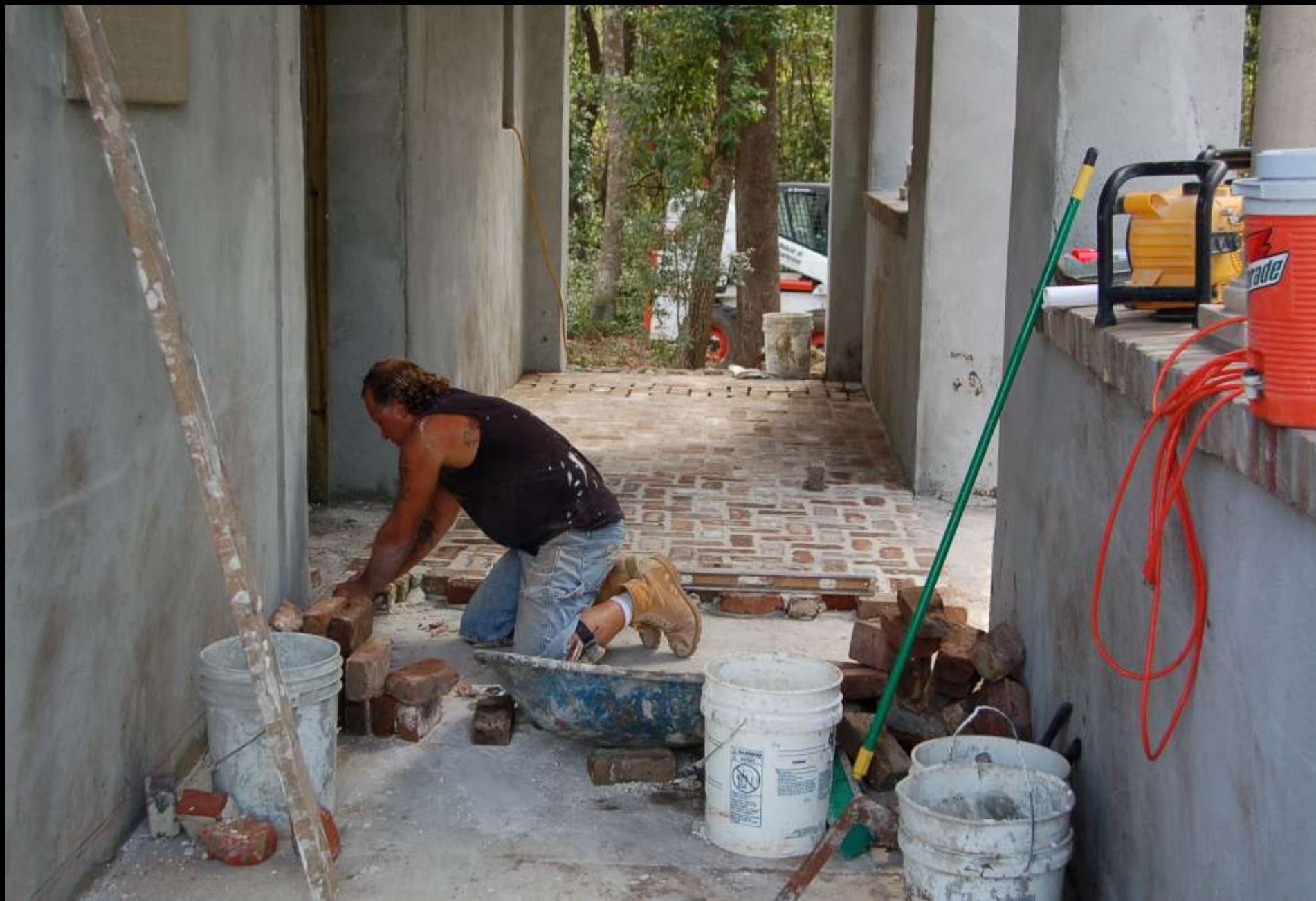
Laying the antique brick paving October, 2007
