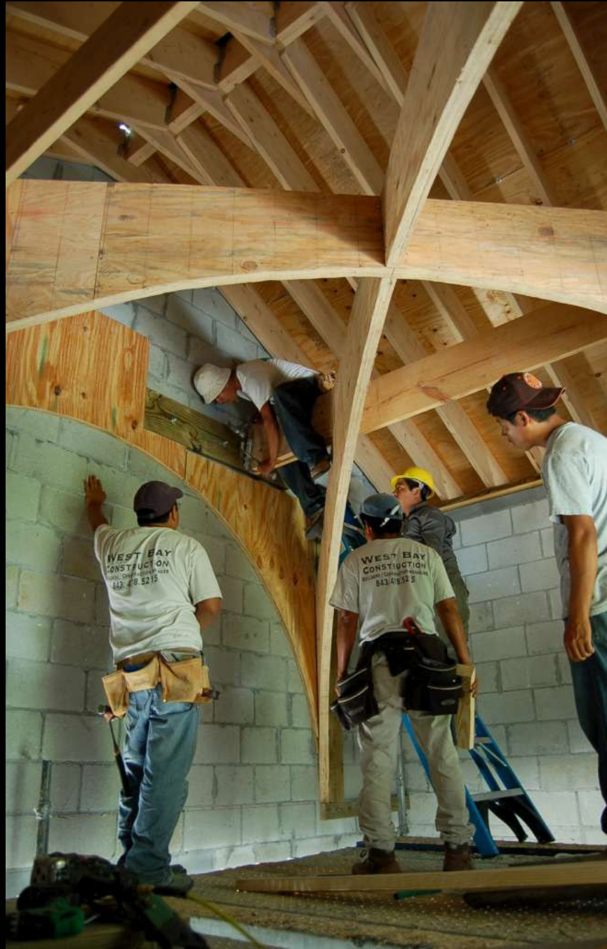
Framing the narthex ceiling April, 2007
