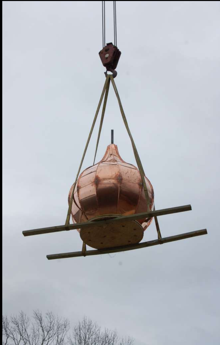
Lifting the first onion dome January, 2008
