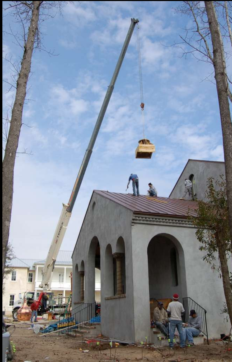
Installing an onion dome base January, 2008
