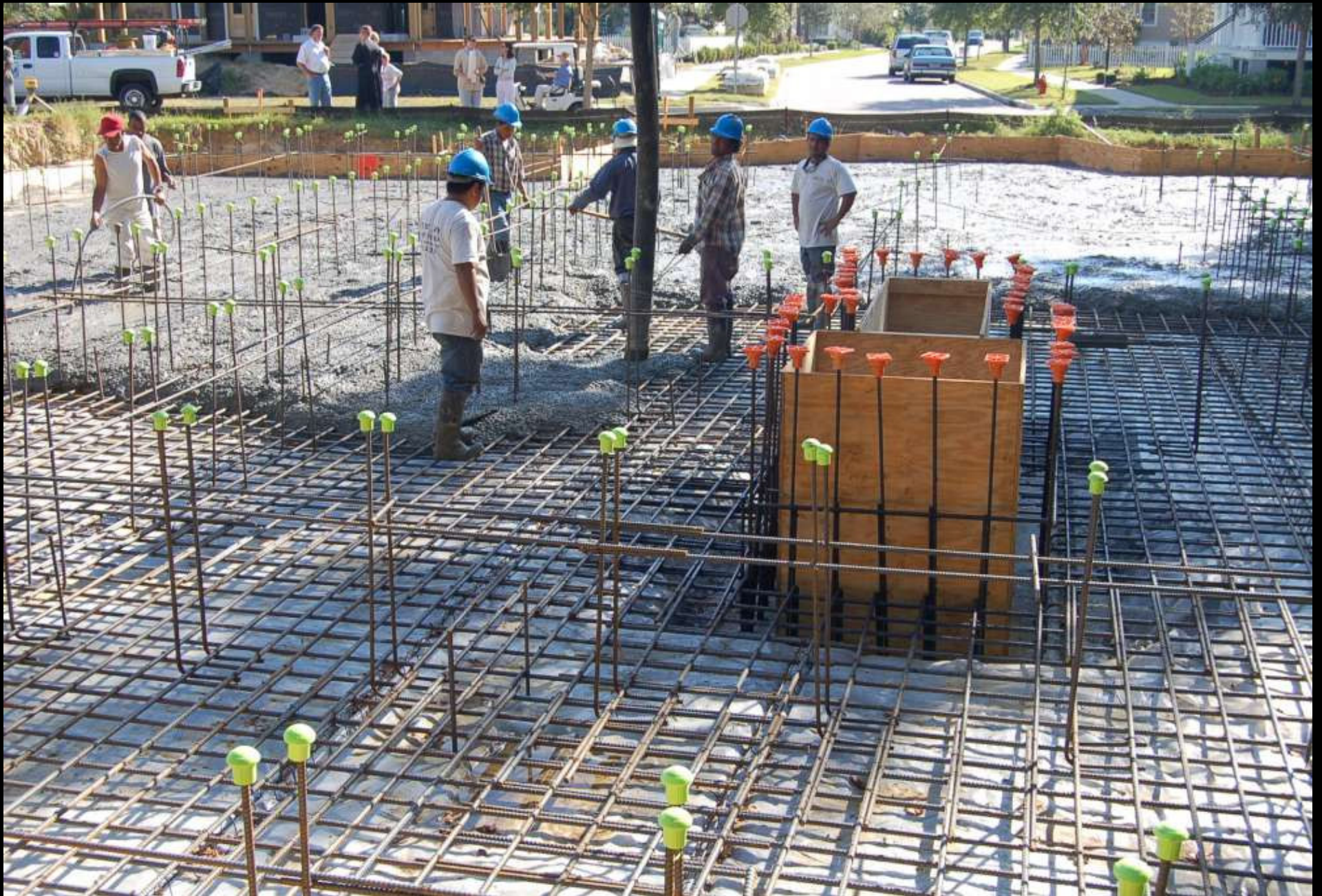
Pouring the foundation slab October, 2006
