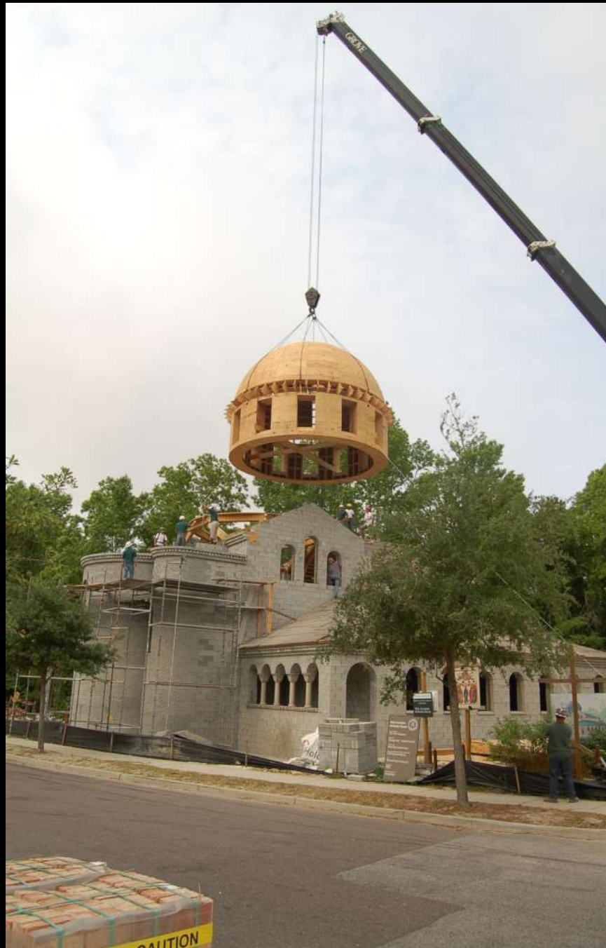
The dome being lifted into place May, 2007
