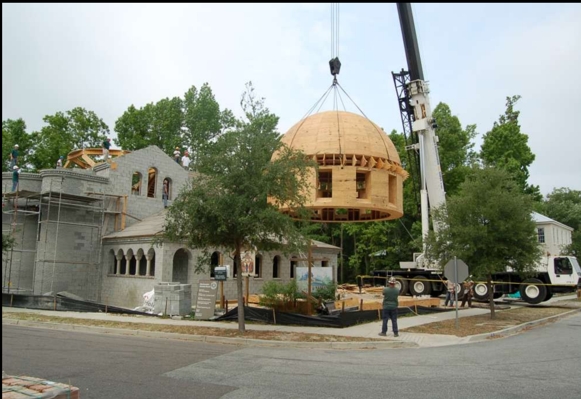
The dome being lifted into place May, 2007
