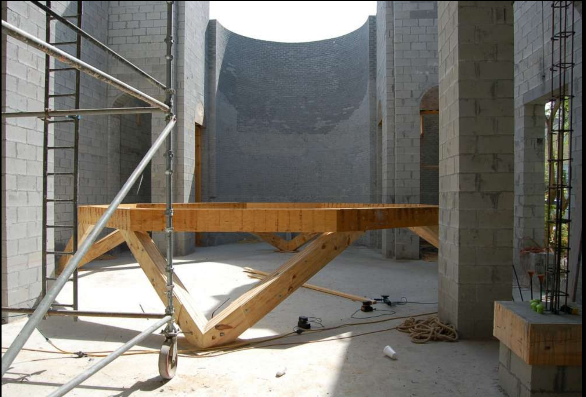
This is the frame which will support the dome April, 2007
