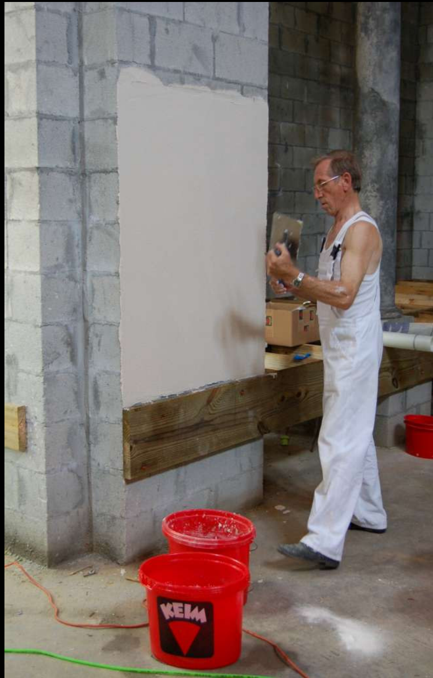
A technical consultant from Germany shows us how to apply the plaster July, 2007
