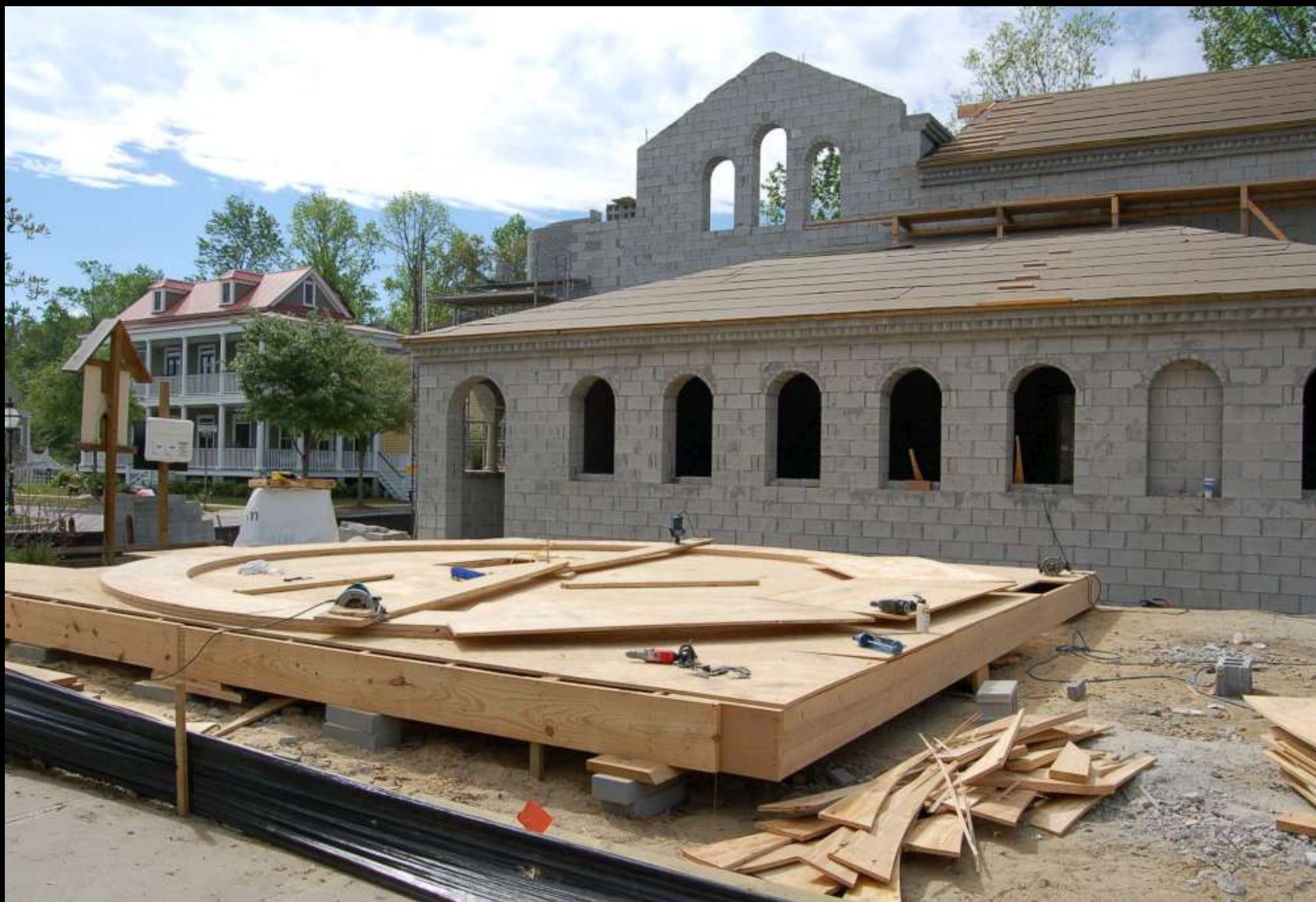
This platform is being used for cutting out the plywood dome ribs April, 2007
