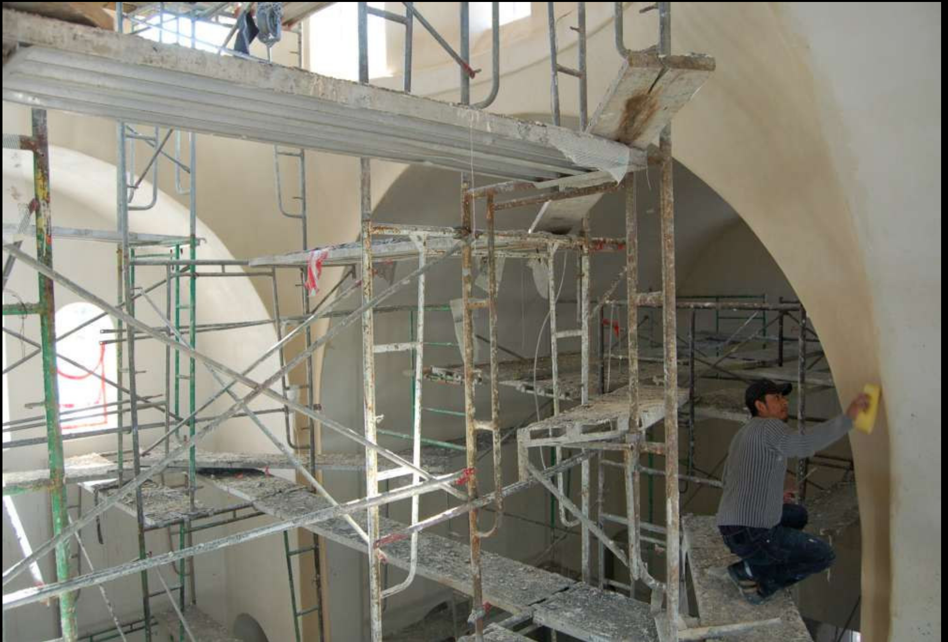
Plastering the interior January, 2008
