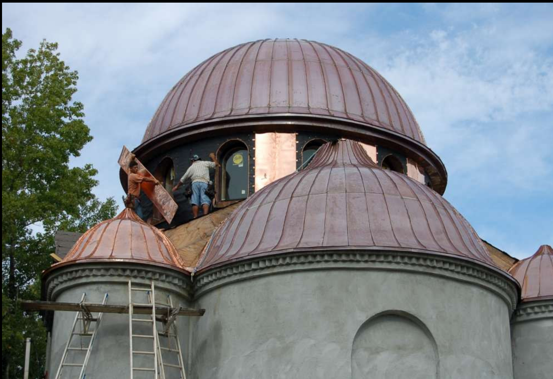
Copper roofing continues September, 2007
