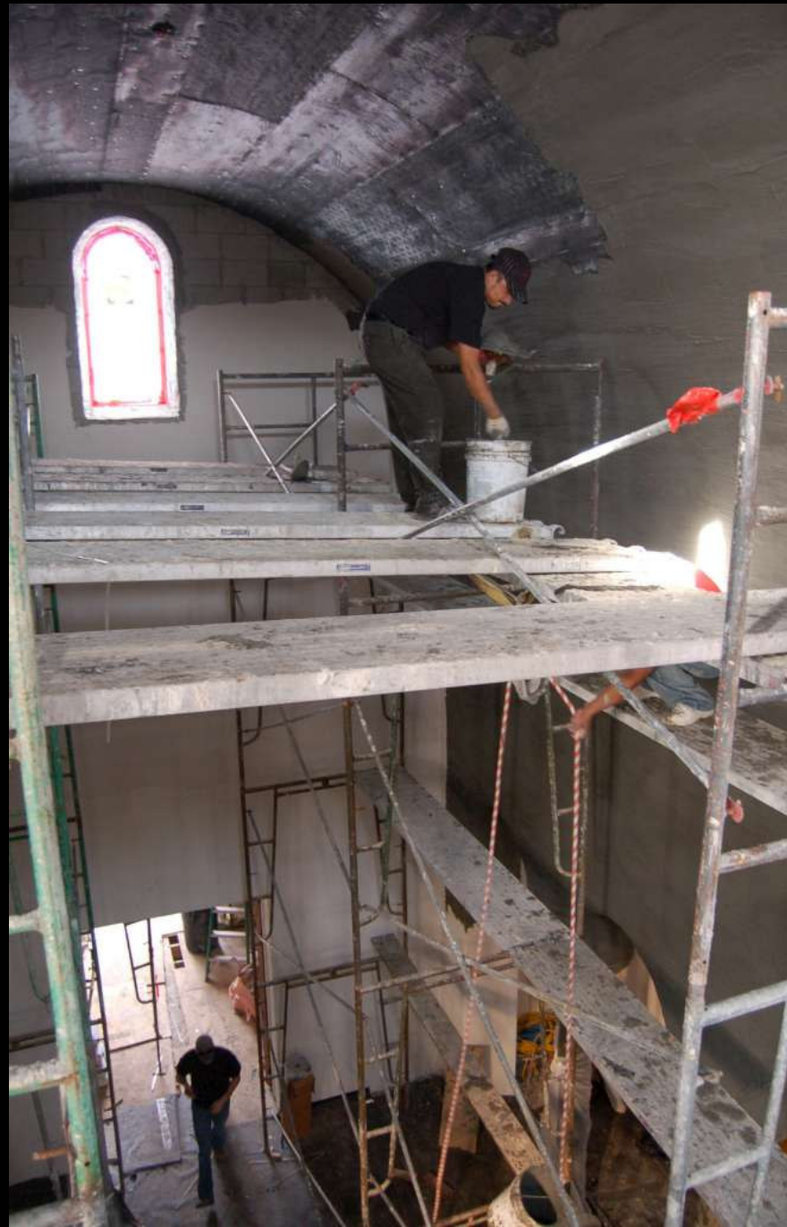
Plastering the interior January, 2008
