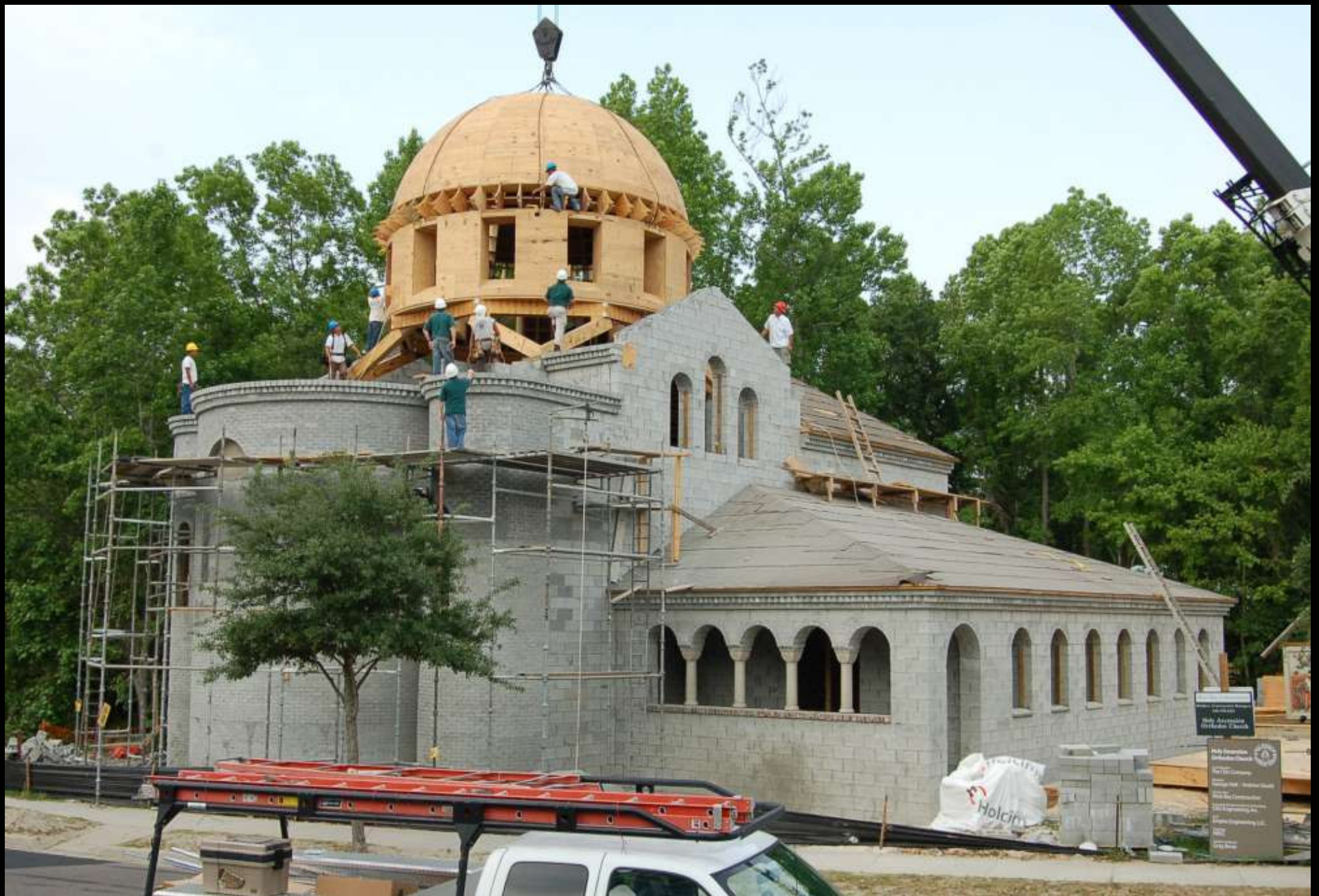
The dome being lifted into place May, 2007
