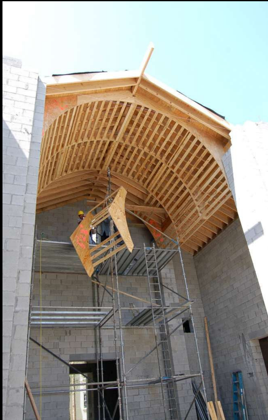
Beginning the vaulted ceiling framing March, 2007
