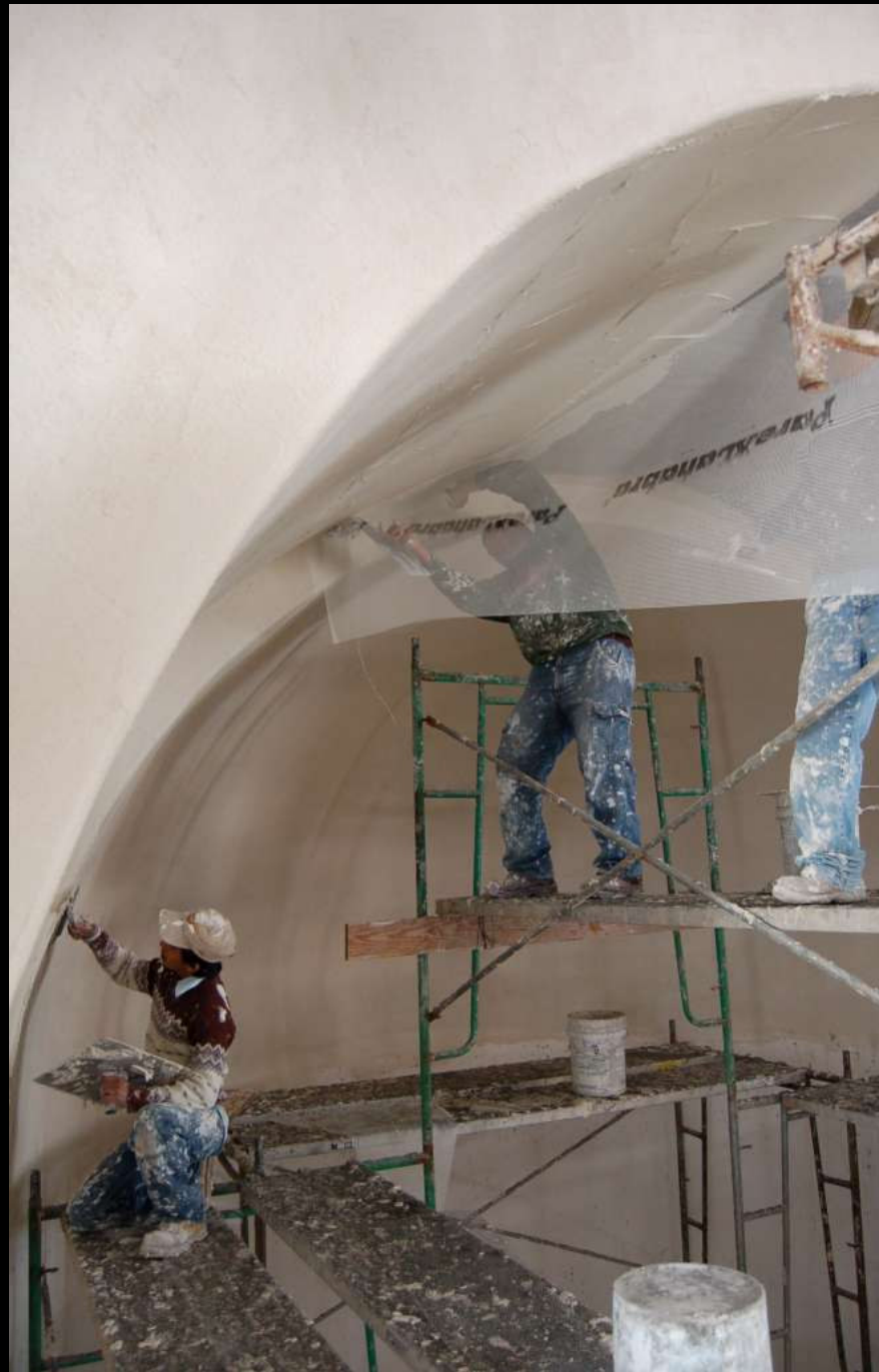
Plastering the interior January, 2008
