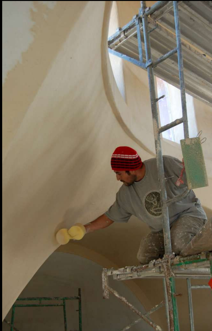
Plastering the interior January, 2008
