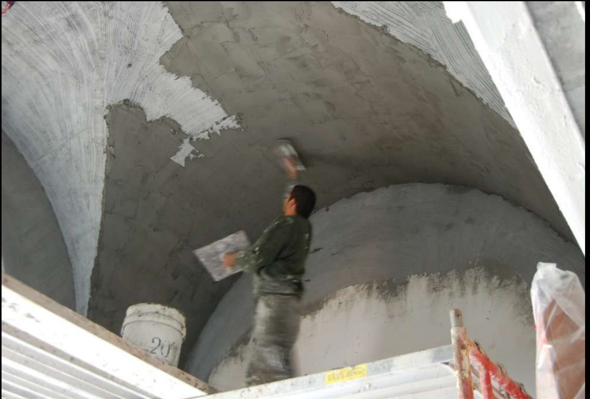
Plastering the interior January, 2008
