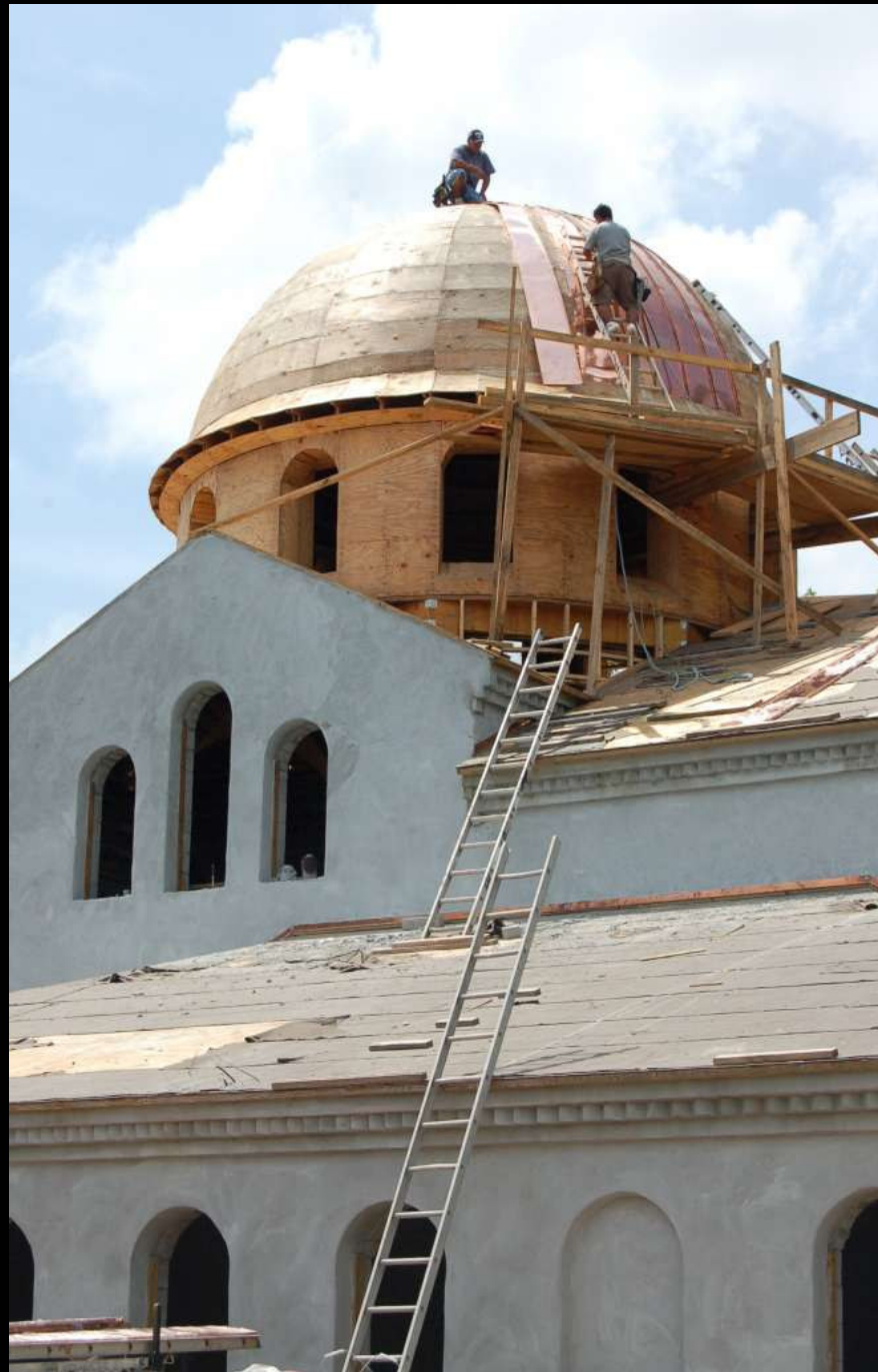
Copper roofing begins on the dome June, 2007
