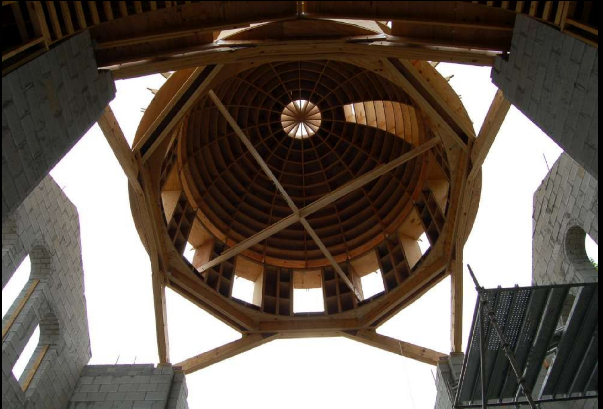
The dome in place resting on the octagonal frame May, 2007
